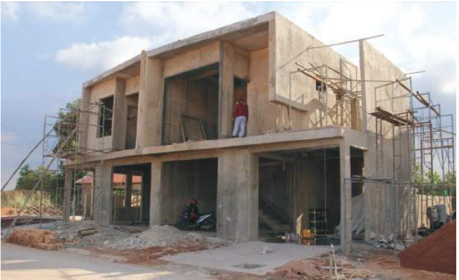
Semi Detached house is on finishing
