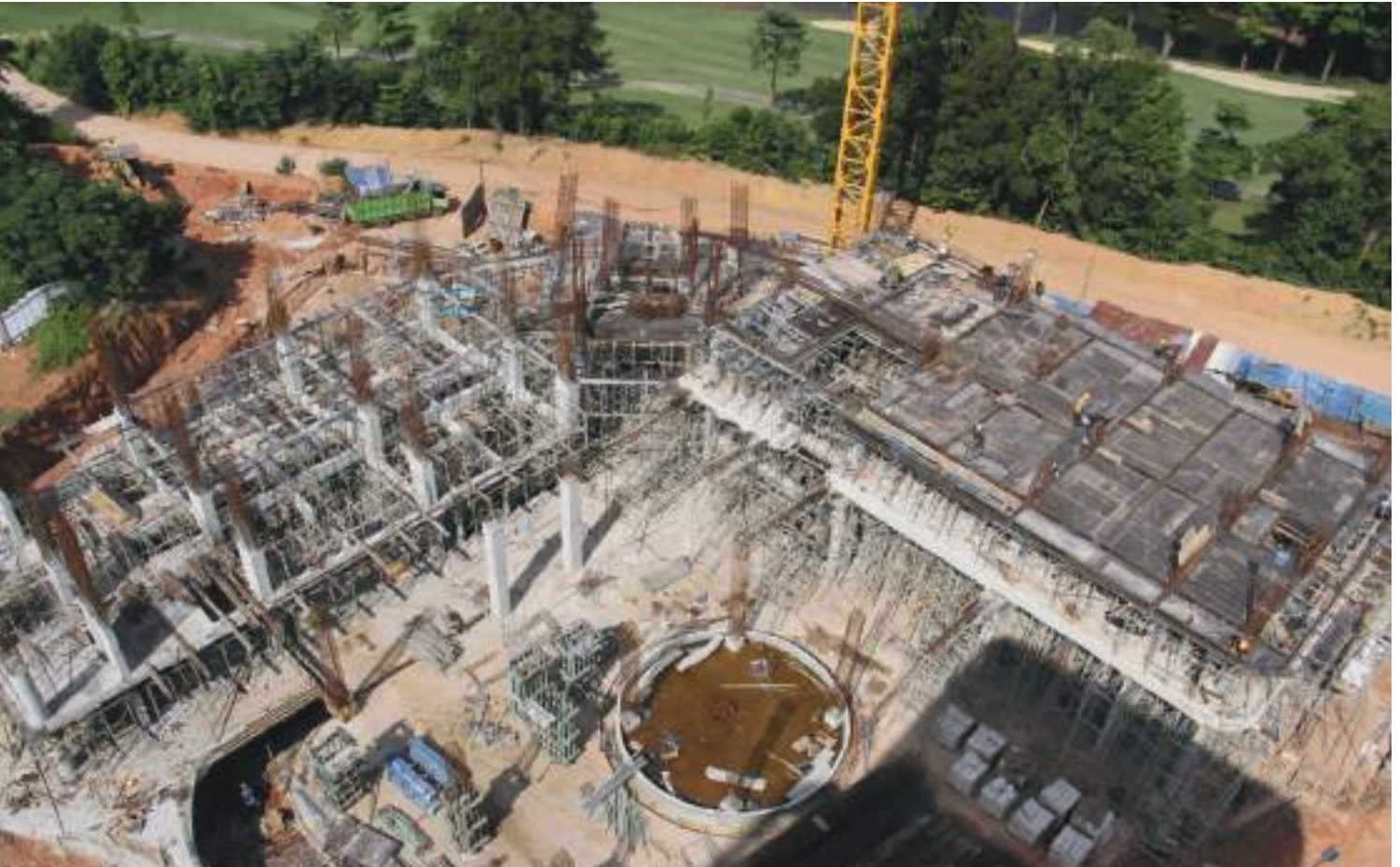
Structure on the third floor, Kalani Tower
