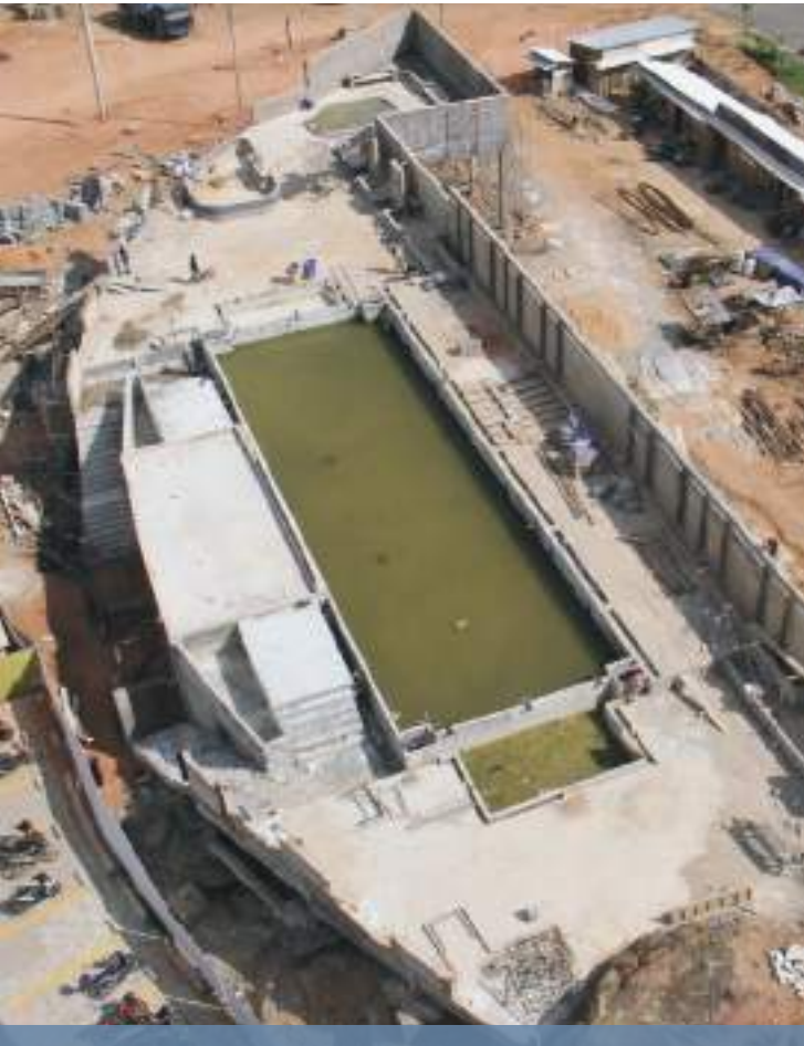
Swimming pool has reached on finishing stage
