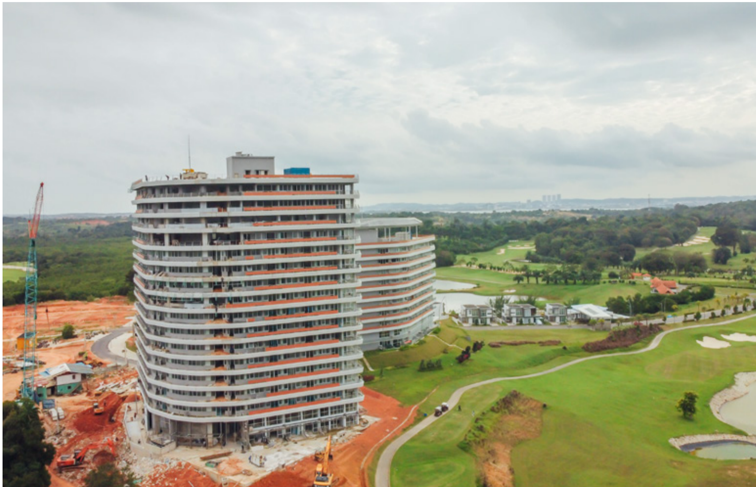
Kalani Tower Construction, The Nove
