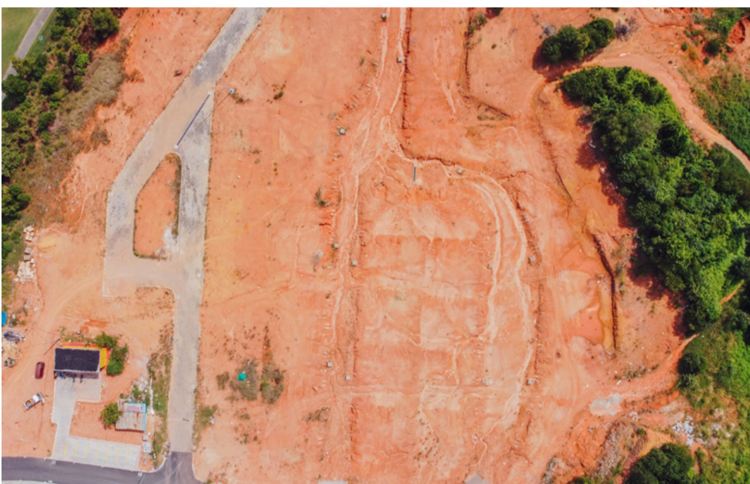
Construction of Landed House phase 2
